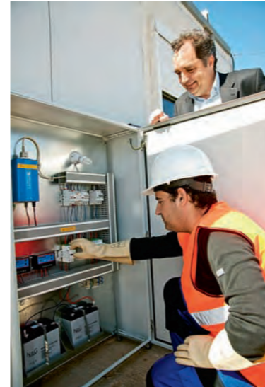
Training programme for installation of photovoltaic systems.
