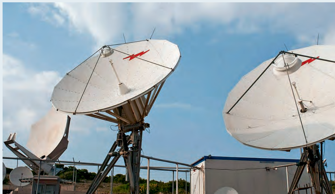
Mechanical engineer D. Karagiannis and chemical engineer A. Gika in the lab of Inasco, an aeronautics company (above). The satellite dishes located on the upper edge of the park transmit TV signals all over the world (on the right). Opposite page: N. Mikroudis of Twin Peak SA showed us a device that offers movies on demand, while I. Arabatzis' Nanophos (right) is one of the most advanced companies in the park.
